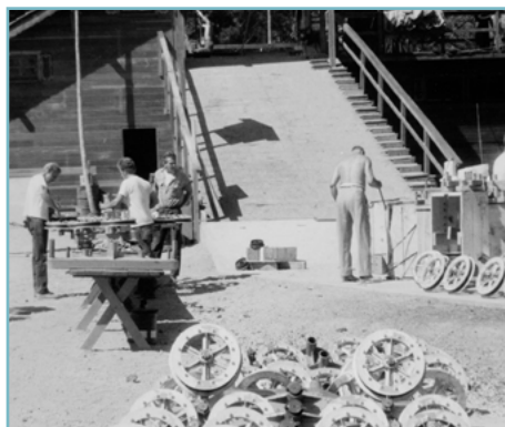
Sheave and sheave assemblies for building Chair 2 in 1957. Original Chair 1 in the background.
