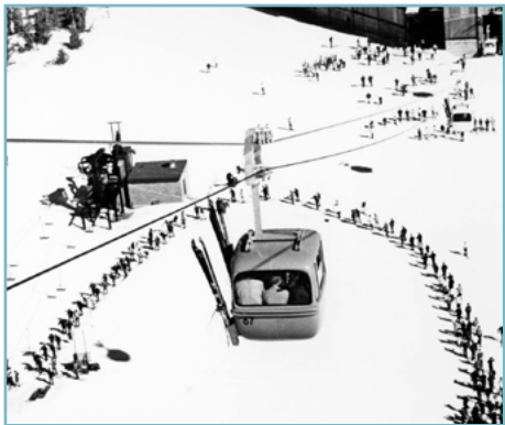
The original gondola was the first of its kind in America, a two-part bi-cable lift. The top cable was the "carrying cable" and did not move. The cabins were connected to the lower cable that is pulled the cabins up the mountain. The top gondola opened in 1967 and allowed lift-served access to some of the best skiing on Mammoth Mountain.
