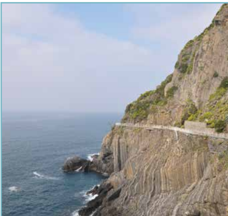
Lower trail from Riomaggiore to Manarola was closed due to rock slides.
