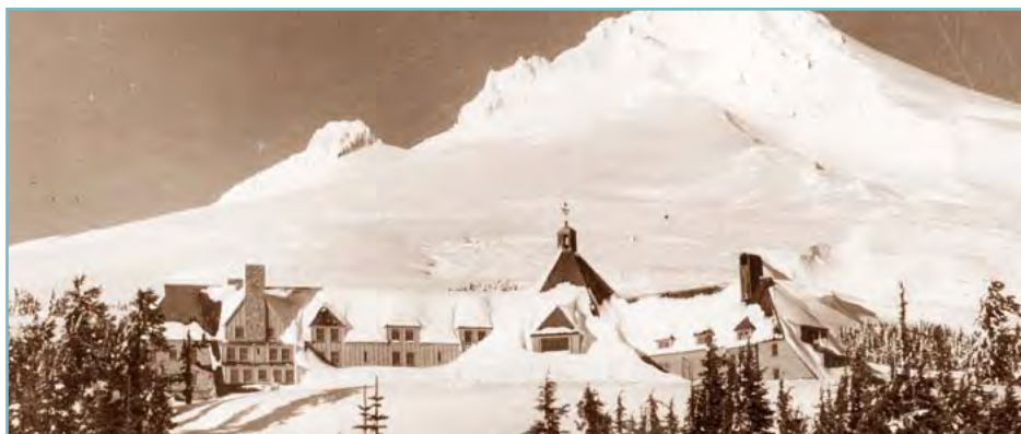
Mt. Hood and Timberline Lodge in 1943.
