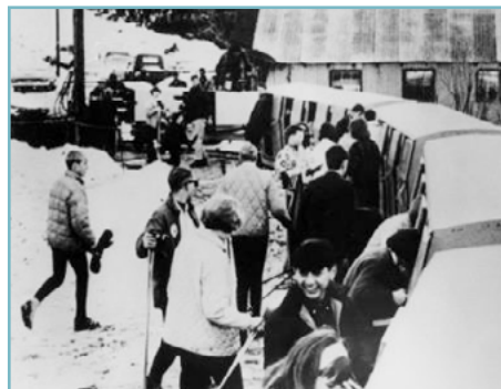
Skier's Subway through Spiro Tunnel.
